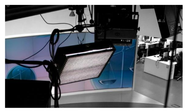
Replacing of all the old lighting of the Antena 3 News set with new LED technology.
