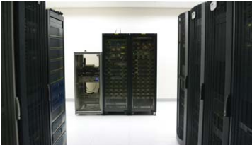
KSA IT Center
