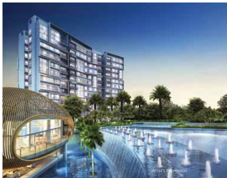
The Palette is well-located near Pasir Ris MRT, amenities and outdoor recreational facilities.
