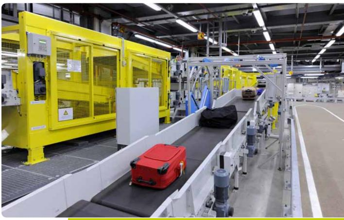
The baggage basements house 21 kilometres of conveyors and a five-kilometre rail system. Schiphol has the most advanced baggage system in the world.
