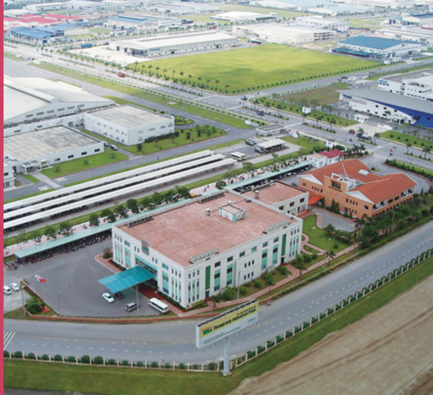
Thang Long Industrial Park in Vietnam
