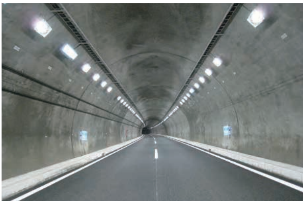
Long-life lighting in tunnel
