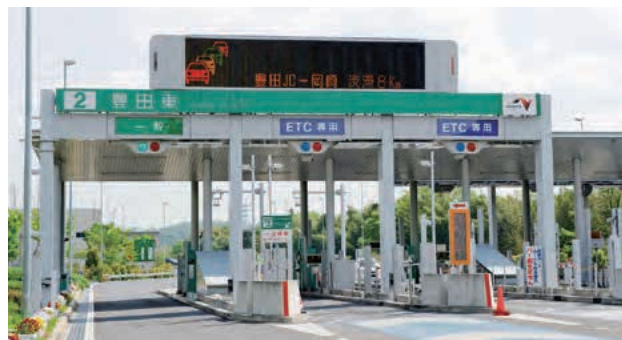
ETC gate at the Toyota-Higashi Interchange on the Ise-Wangan Expressway
