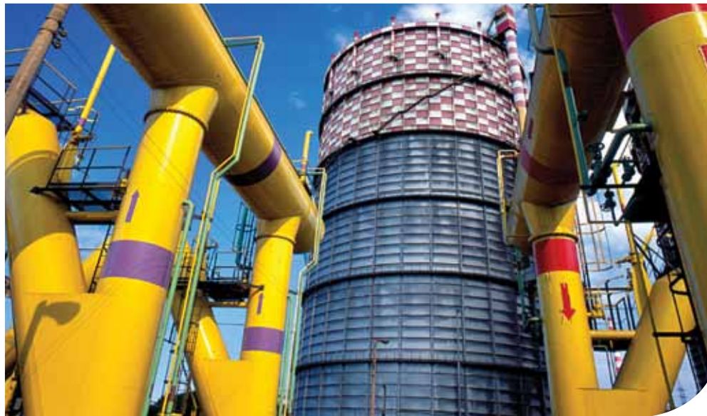
Gas meter in Tubarão: reuse of gases guarantees energy self-sufficiency
