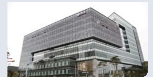
A Picture of the Group’s Integrated Data Center
