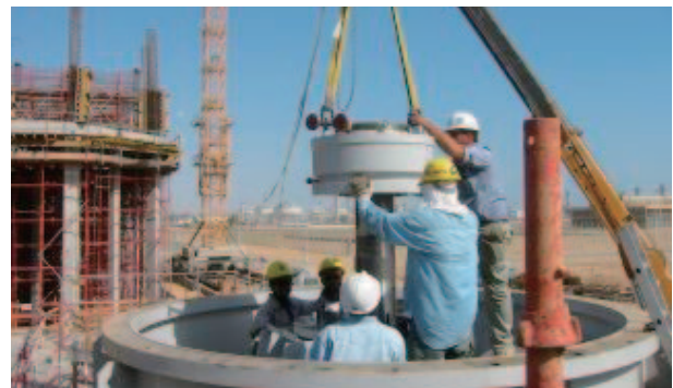
Supervision of the assembly of a duplex stainless steel seawater pump (Saudi Arabia)
