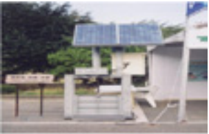
Photovoltaic-powered gate installed to reduce energy consumption for business operations
