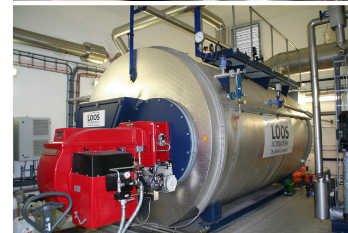
Top: Co-workers Mats Ivar Kjønnøy and Ståle Breivik monitor the production process at GC Rieber Oil’s production plant in Kristiansund, Norway. Above: The new steam boiler where bio diesel now has replaced fossil fuel.
