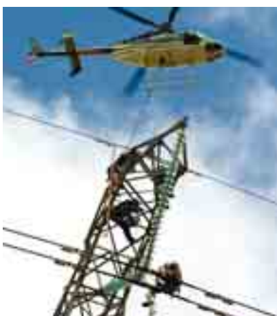
Liveline team replacing insulators
