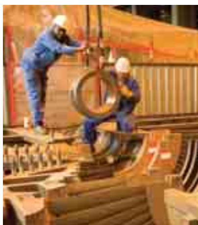
Camden power station refurbishment in progress
