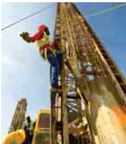
Construction being carried out at Atlantis open cycle gas turbine site
