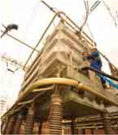
Maintenance work being carried out at Apollo substation
