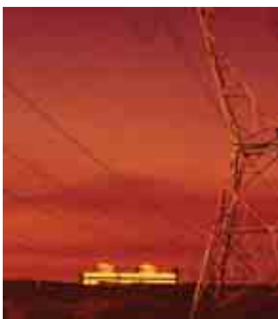
Koeberg power station feeds into the national transmission grid
