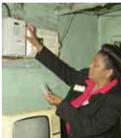
Demonstrating a prepaid meter to a newly electrified customer
