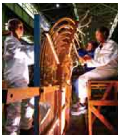
Re-taping the harness of a high voltage transformer at Rotek
