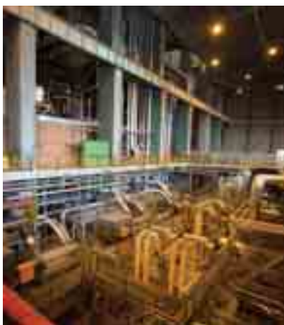
Recommissioning in progress on the generation floor at Camden power station
