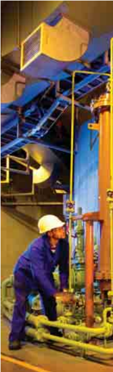
Routine maintenance at Palmiet pumped storage scheme
