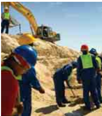
Foundation work at Atlantis open cycle gas turbine site
