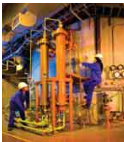
Routine maintenance at the Palmiet pumped storage scheme
