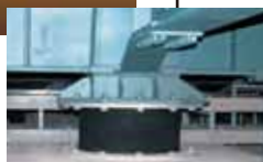
Seismic Isolator
