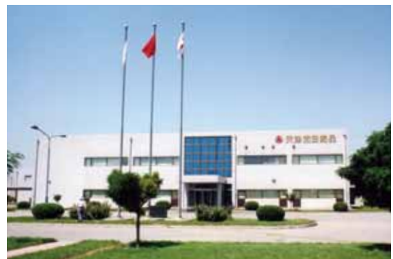
Tianjin Takeda plant
