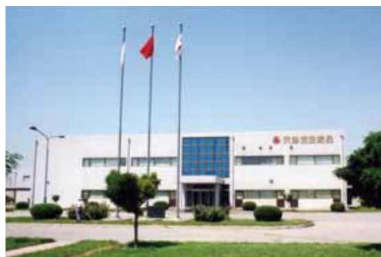
Tianjin Takeda plant
