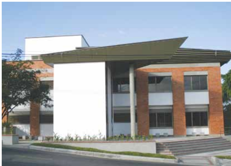
Cold Cuts Business R&D+i Center
