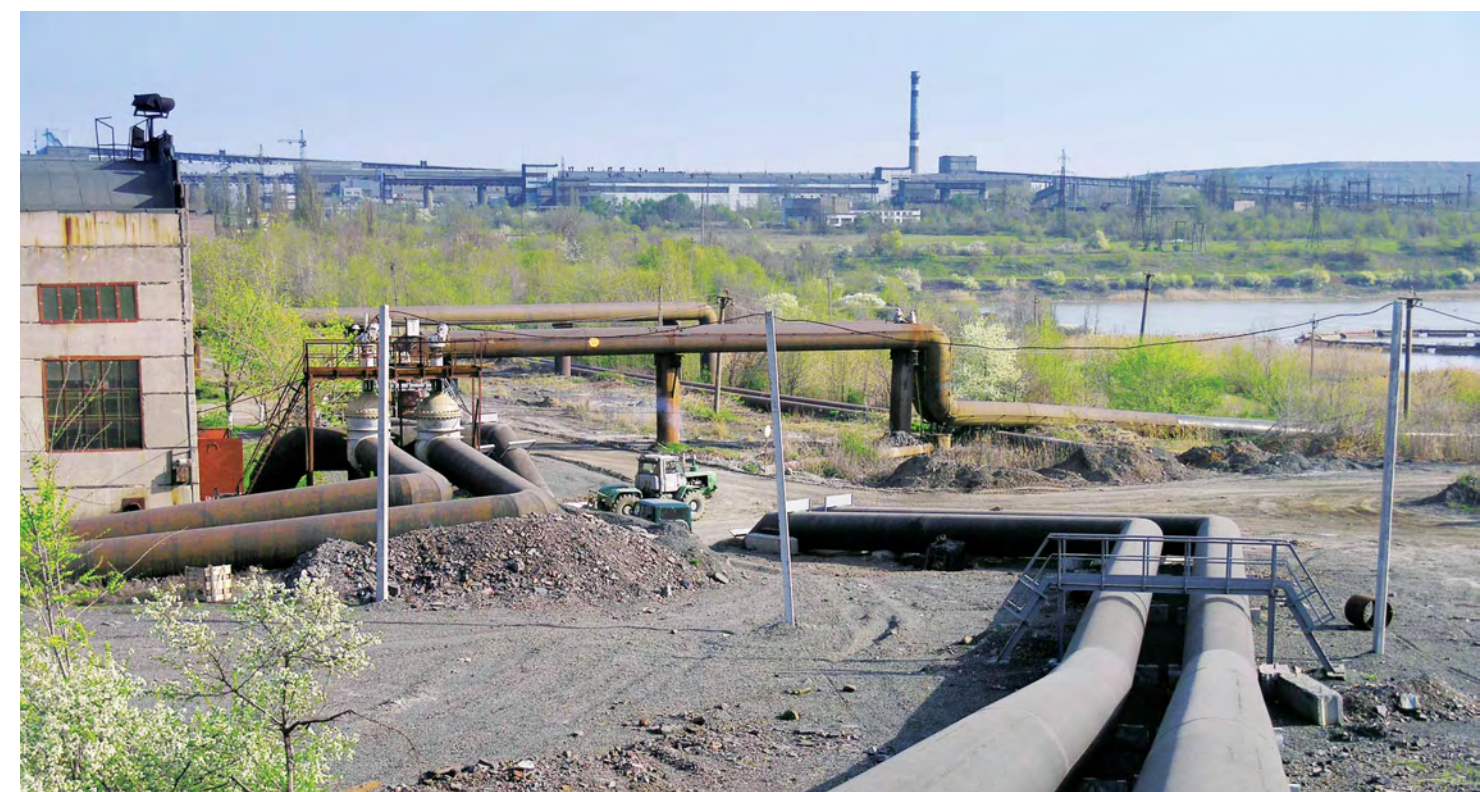
Construction of two gravity water conduits to supply process water to the ore preparation plant in Ingulets GOK
