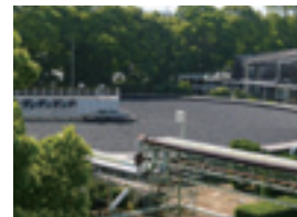
Sedimentation tank before improvement
