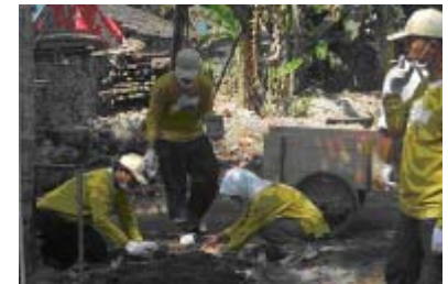
Rehabilitation of disaster area in Bantul, Yogyakarta, 2007
