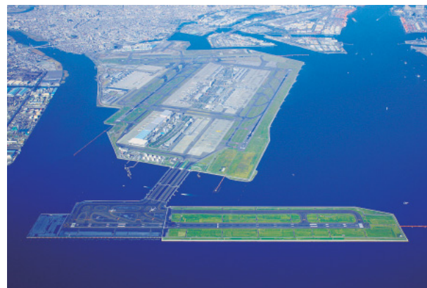
The newly opened Runway D at Haneda Airport (Haneda Airport Expansion Project JV)
