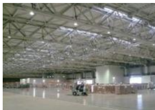
A completely pillar-less structure ensures the shortest, optimal lines of movement.
