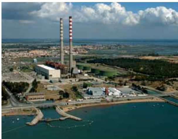
Setúbal Thermoelectric Power Station
