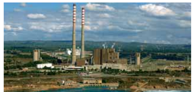
Sines Thermoelectric Power Station
