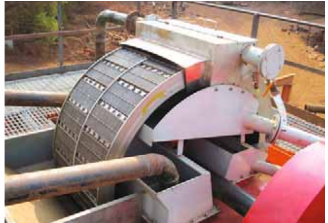
WHIMS installed at Codli
