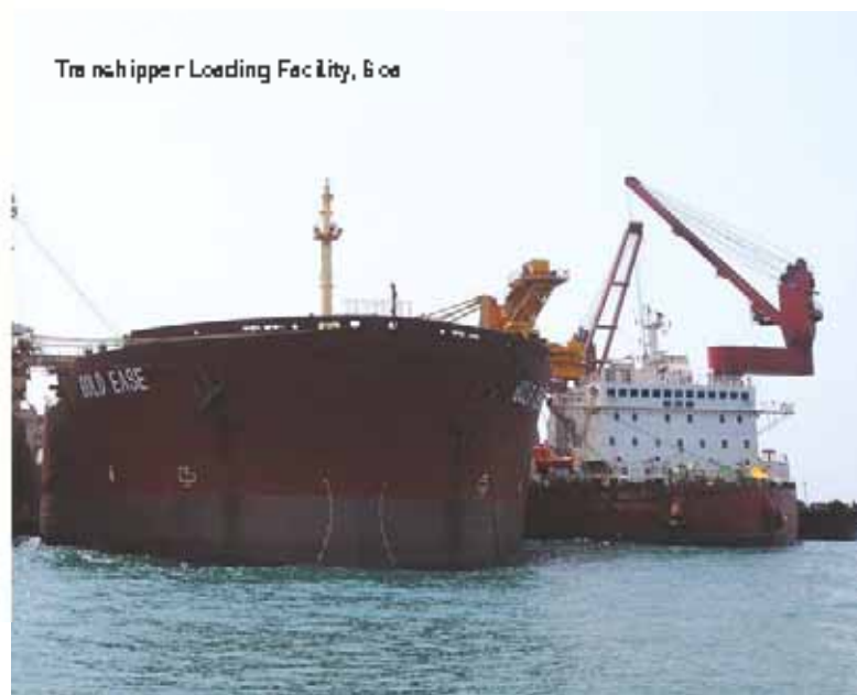
Transhipper Loading Facility, Goa
