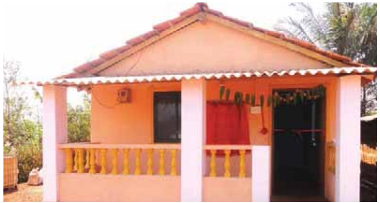
House constructed for underprivileged at Amona
