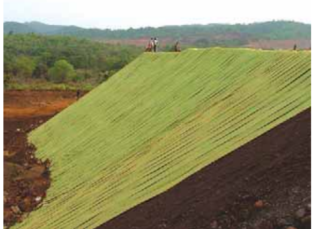
Laying of Geotextile at Codli Mine
