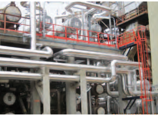
Detail of the crude heat exchanger train of the La Rábida refinery, the energy improvement of which was developed by OHL Industrial and has merited Customer recognition.
