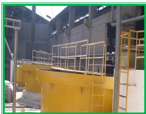
Clarifier of Effluent Treatment Plant
