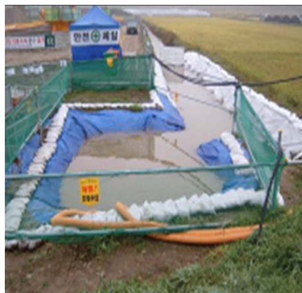
[Installing a Temporary Grit Chamber]
