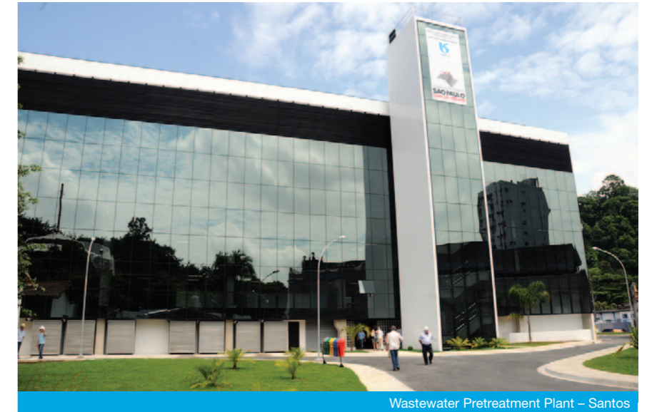
Wastewater Pretreatment Plant – Santos
