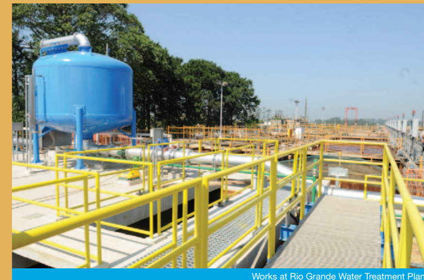
Works at Rio Grande Water Treatment Plant
