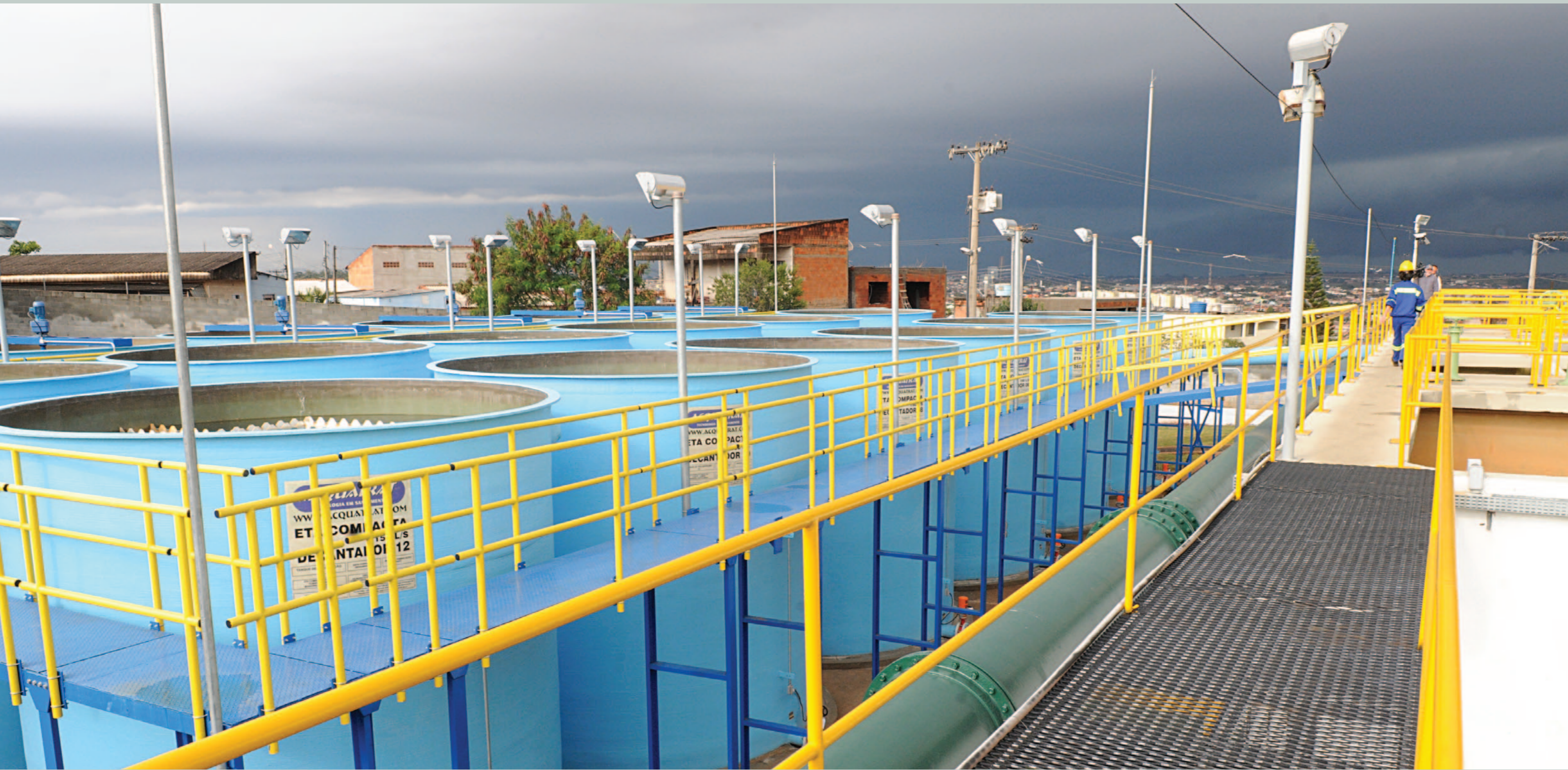
Sumaré Water Treatment Plant
