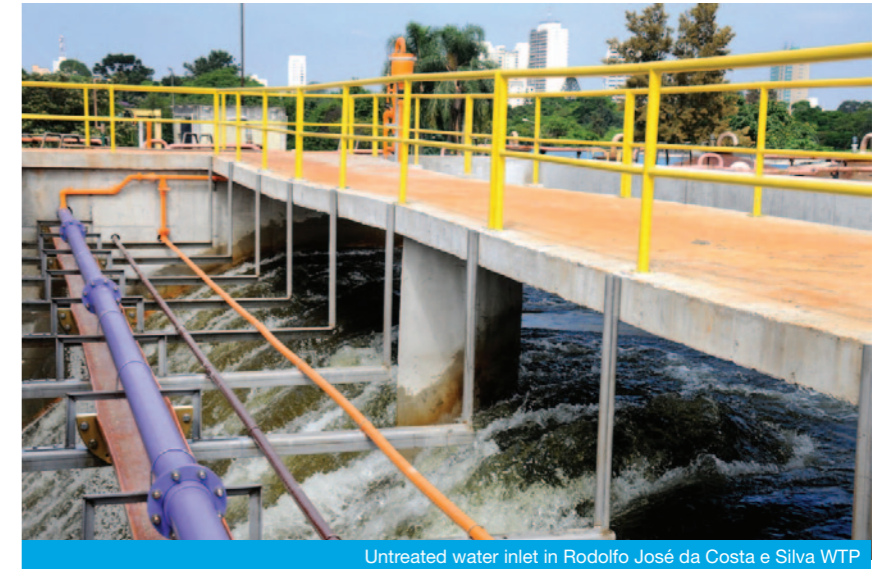
Untreated water inlet in Rodolfo José da Costa e Silva WTP
