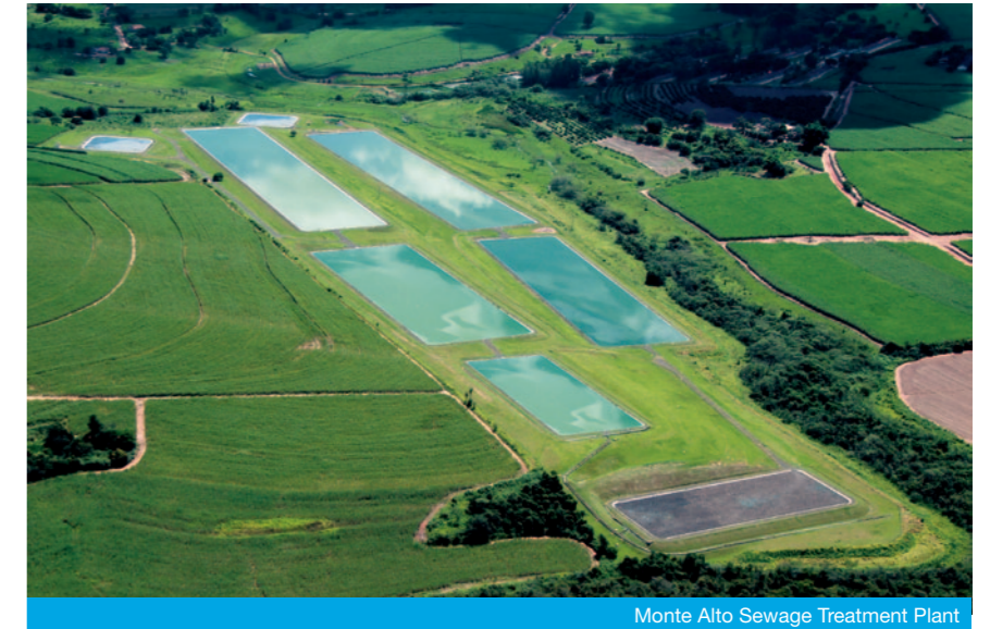
Monte Alto Sewage Treatment Plant
