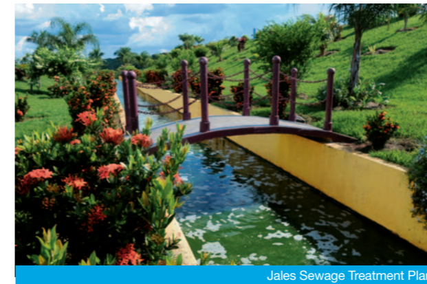
Jales Sewage Treatment Plant
