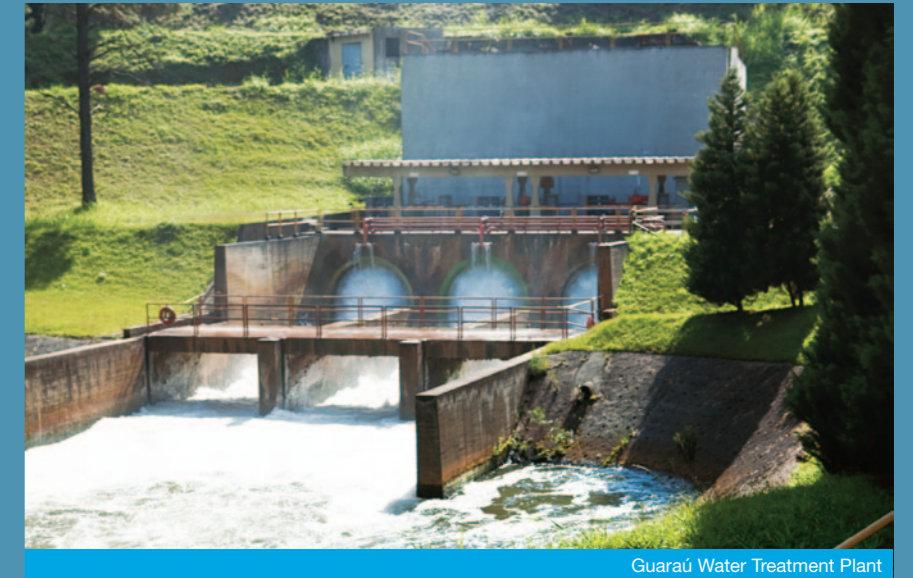
Guaraú Water Treatment Plant
