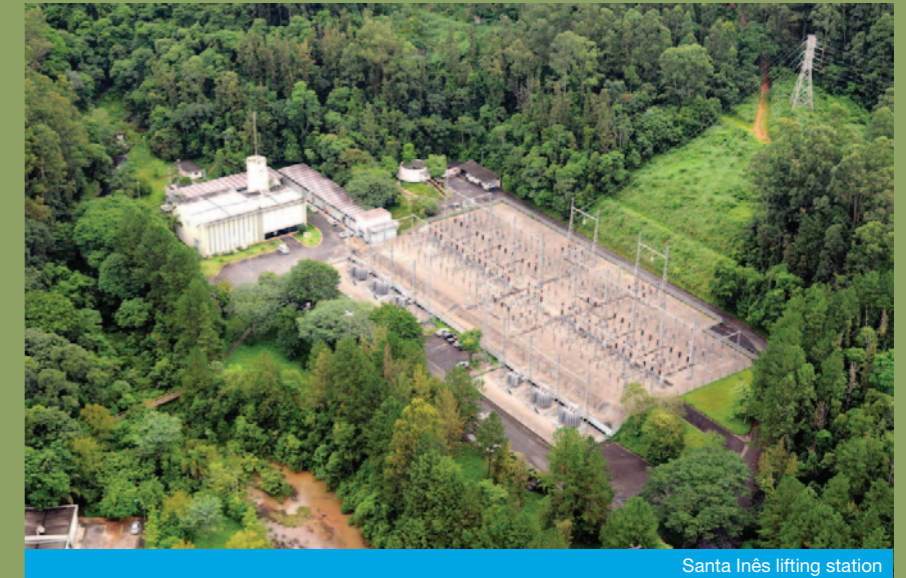
Santa Inês lifting station
