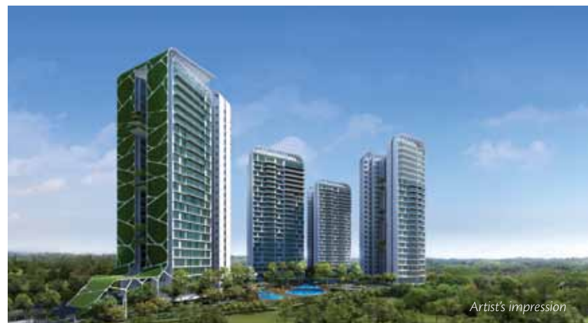
Designed as a green oasis, the numerous green innovations at Tree House is expected to result in energy savings of over 2,442,347 kWh per year and total water savings of 28,968.22 m 3 per year.
