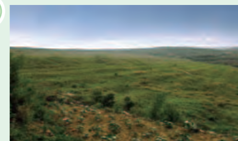
Tailings dam with restored vegetation
