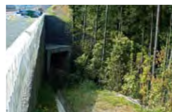
Embankment with a retaining wall
