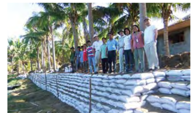
Embankment made with sandbags
