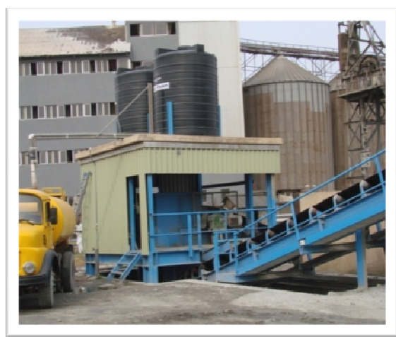
Plate 46: New transfer house at the transfer point between number 2 and 3 conveyors.
