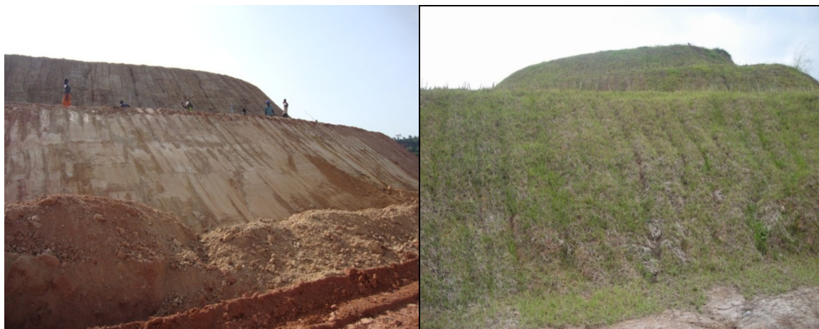
Plate 21:shows newly constructed footwall slope
