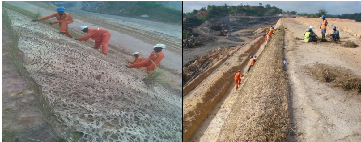
Plate 25 shows: Spreading of jute mats
