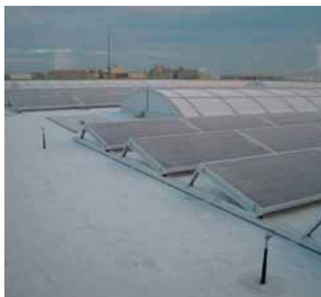
Installation of photovoltaic panels on the warehouses at DP World Breakbulk in Antwerp, financed by Dexia as part of its Dexia Energy Line – Renewable Energy offering
