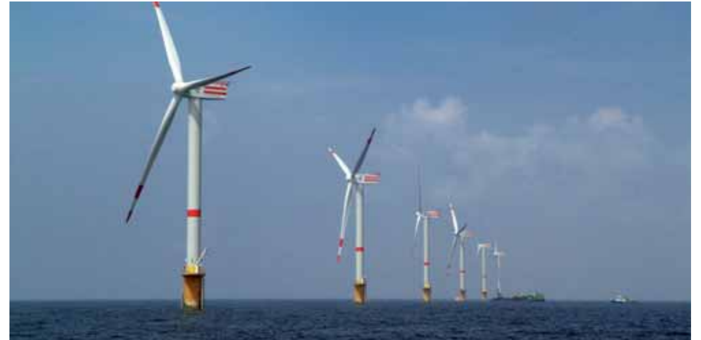
C-Power, Belgium's first offshore wind farm
