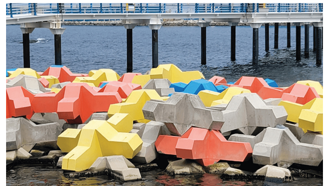
Marine construction utilizing pond ash (Sofa block)
