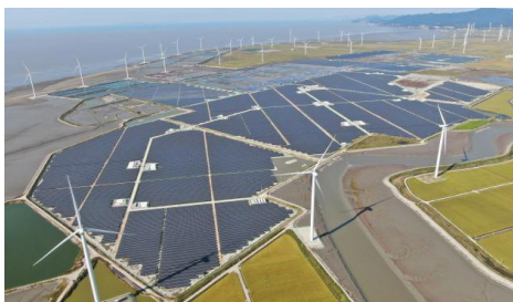
Solar power generation complex using an abandoned saltern
