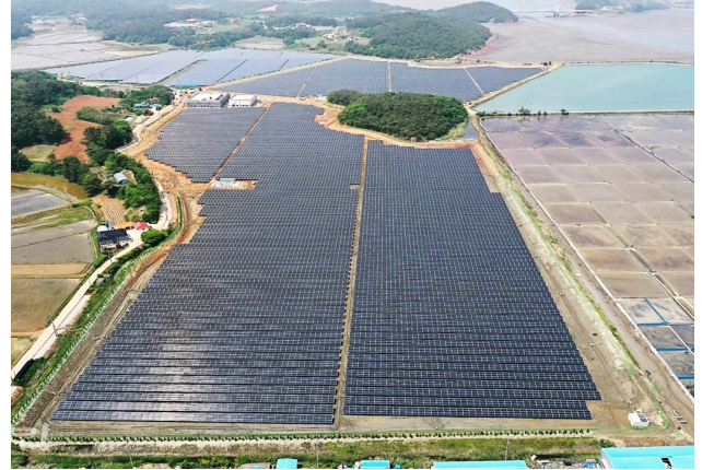
KOWEPO | Construction of Solar Power Generation in idle sites
