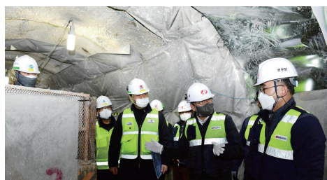
Special Safety Inspection on Construction Site by CEO
