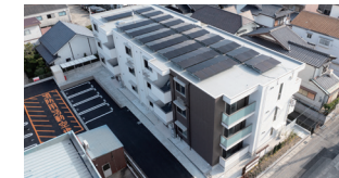
A ZEH-M compliant rental housing
