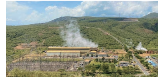
Olkaria II Power Station
