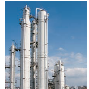
ENEOS Materials chemical plant (former JSR chemical plant)
