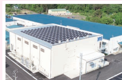
Precision metal mold building
