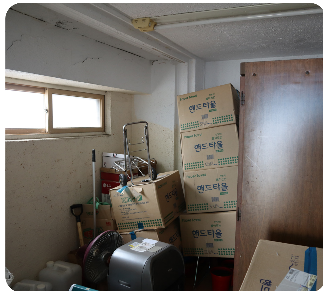
Graceful Shelter: Before renovations
