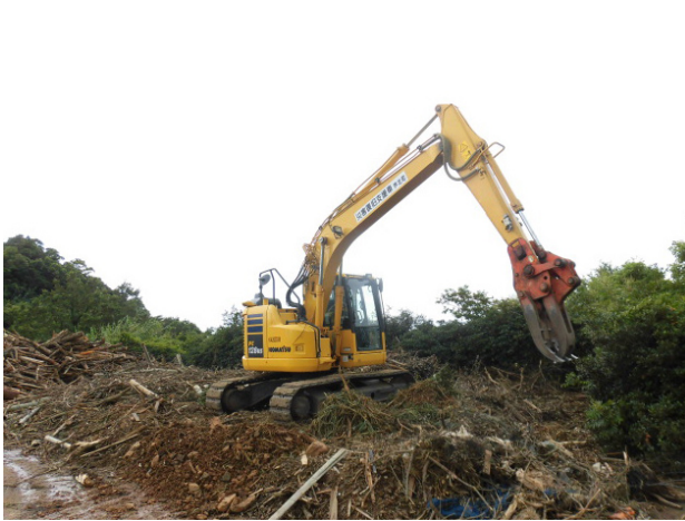
Clearing driftwood in Ashikita Town
