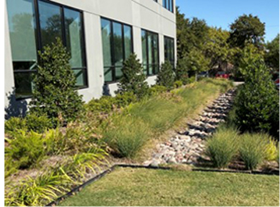
Hensley's Dallas facility : Bioswale
