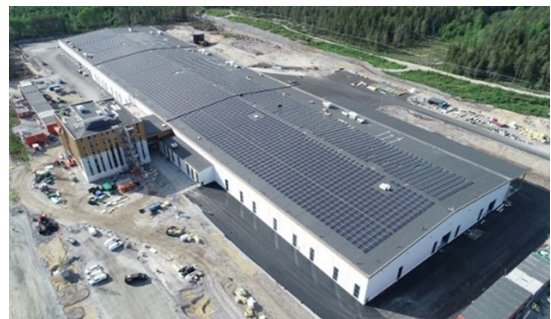
Solar panels of the new plant
