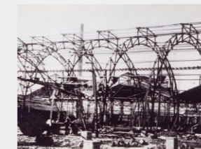
Fukagawa Plant being rebuilt following damage in WW2
