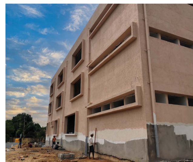
The Skill Development Training Centre is a state-of-the-art facility equipped to train students with disabilities.
