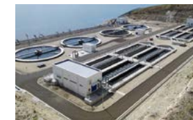
Sewage treatment plant
