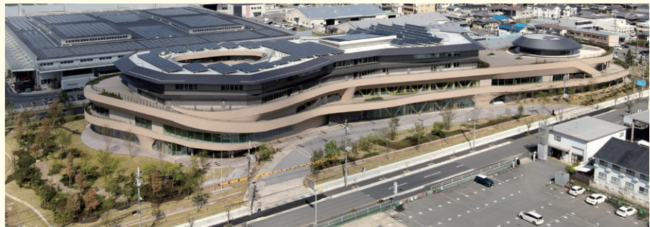
Our Group's a new training facility, the Daiwa House Group MIRAI KACHI KYOSO Center in Nara embodies the ZEB concept
