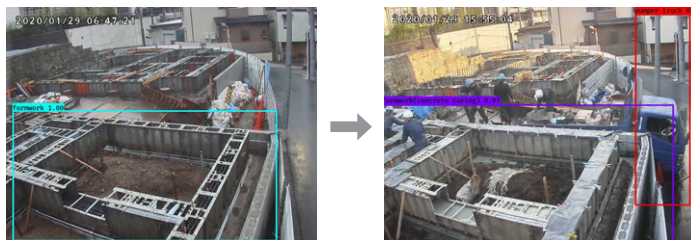
AI monitors construction progress based on images from camera
