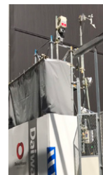
Scene of installation
