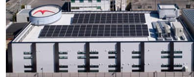
Approximately 120 solar panels installed (output: 36 kW)
