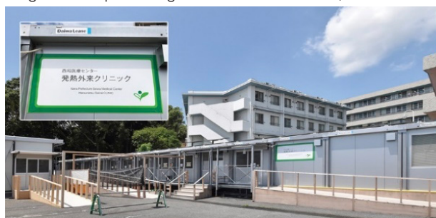
Appearance of the outpatient clinic at Nara Prefecture Seiwa Medical Center
