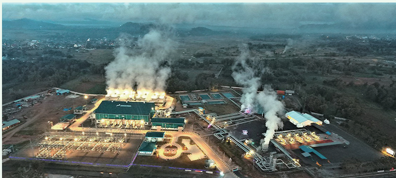
The Lahendong geothermal power plant
