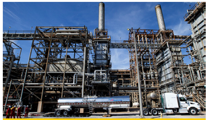
The Shell Norco Manufacturing Complex in the USA uses liquid feedstock made from plastic waste to make chemicals.
