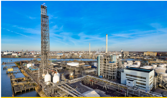
We may use flaring at facilities, such as our Pernis refinery in the Netherlands, if required to safely relieve production system pressure.
