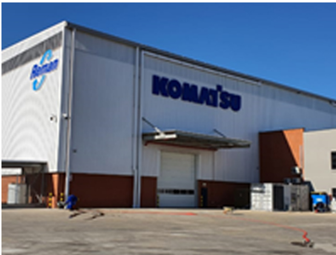
Komatsu Africa Holdings' new Reman building
