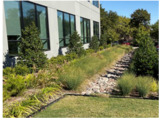
Hensley's Dallas facility : Bioswale
