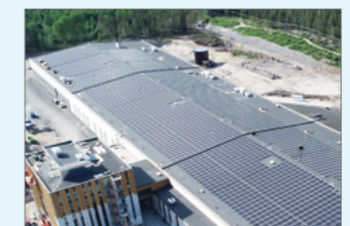
New Komatsu Forest AB factory with roof covered in solar panels (scheduled to be completed in August 2021 in Umeå, Sweden)
