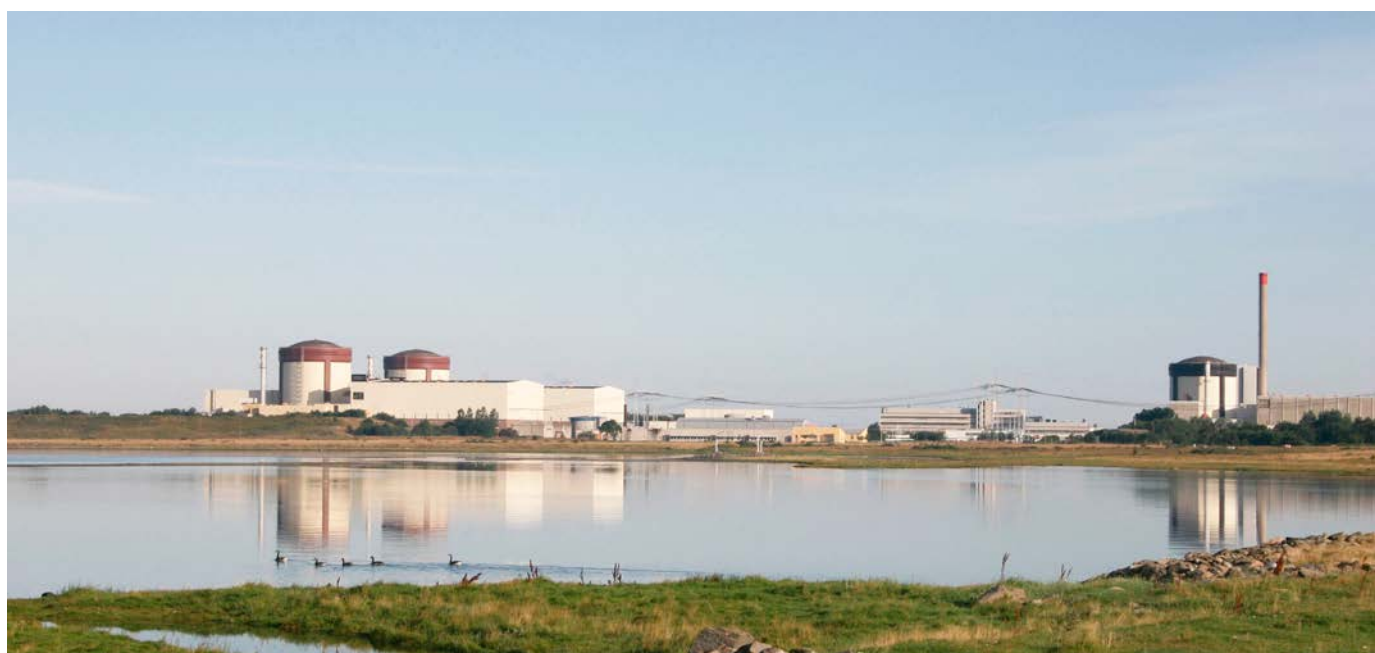
Ringhals 1 left the electricity grid on 31 December.
