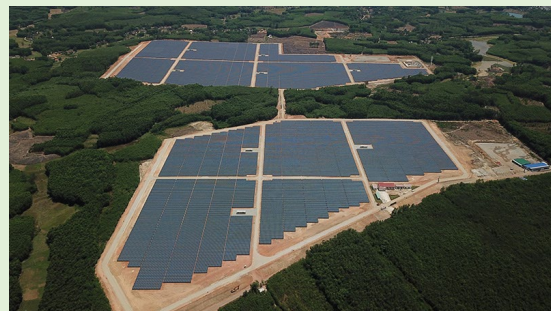
The mega solar power plant is well into operation
