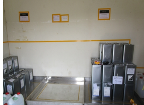
A yellow line drawn to visualize the allowable stacking height of containers in a hazardous material storage area
