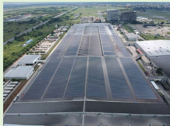
Yokohama Rubber tire factory
