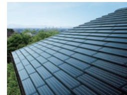
Solar power generation system
