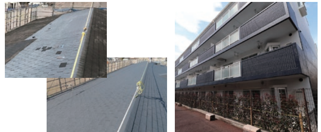
Roof shingle replacement work
