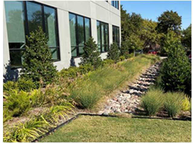
Hensley's Dallas facility : Bioswale
