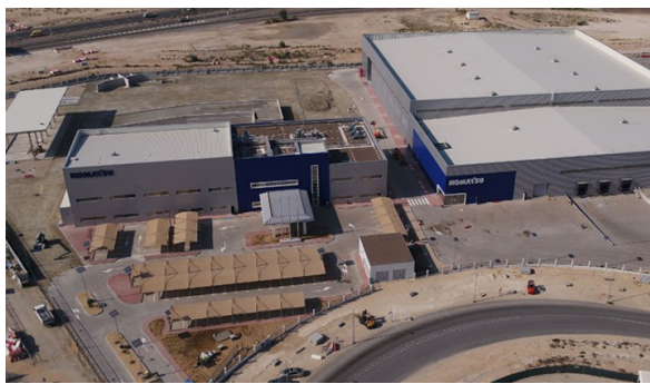
The Dubai Training & Demonstration Center
