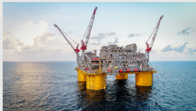
Installing a more efficient power plant at the Appomattox deep-water oil and gas project in the USA has helped cut fuel consumption by around 40% and air emissions by about 20-25%.
