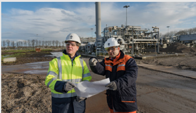
Safe and responsible decommissioning of surface infrastructure at gas production facilities is a priority for NAM.
