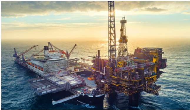
The Brent Bravo platform topside was removed by the Pioneering Spirit, a ship stretching the length of six jumbo jets.
