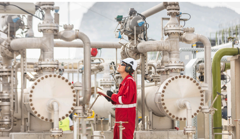
In Gibraltar, we opened an LNG regasification terminal to supply the territory's new gas-fired power station.
